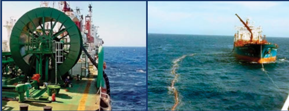
Fig. 2. Offloading operations via flex hose to a shuttle tanker.
